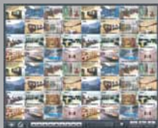
central monitoring system (CMS)
